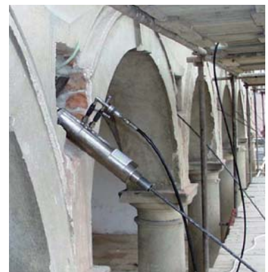
Repair of vaults of baroque colonnade
